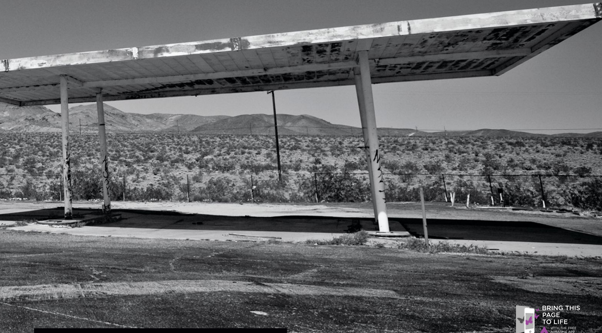
ABANDONED GAS STATION. ROUTE 66, MOJAVE DESERT, CALIFORNIA
